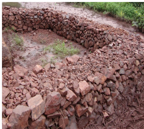
Pic-7: Check weir along the nallah
