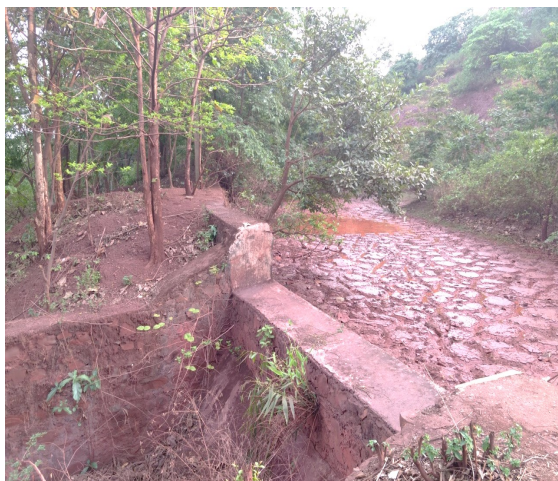
Pic-3: Settling Pond & Check Dam
